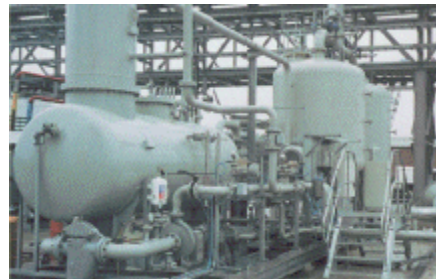
Vapour recovery unit (VRU) installation
