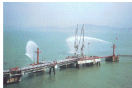
Fuel Jetty at Chek Lap Kok Airport, Hong Kong Parsons Brinckerhoff/ Trident J.V. provided design services for the on-airport aviation fuel receipt, (Fuel Jetty & Pipeline) Tank Farm distribution pipelines and fuel hydrant installation.
