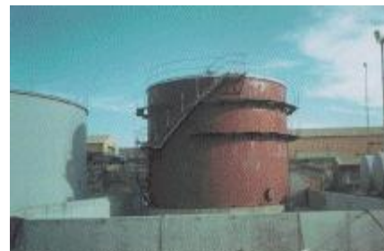
Stanley Services Ltd, Falkland Islands expansion of storage facilities.
