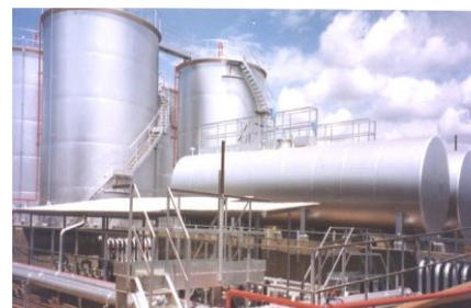
Moshi, Tanzania Terminal re-development
